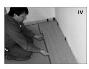
in length (III). Continue the second row with a full piece, placing the tongue of the long side into the groove
