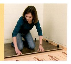
For applications where solid-wood acoustics are important, our Safe&Sound Underlay provides the sound transformation you need. In addition to its unique acoustic properties, Safe&Sound also offers antimicrobial protection against mold and mildew. Its moisture and vapour protection makes Safe&Sound ideal for basements, bathrooms and general, over-concrete installations.
